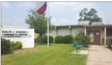
EVELYN CHURCHILL COMMUNITY CENTER in Galena Manor is now closed for remediation work.
