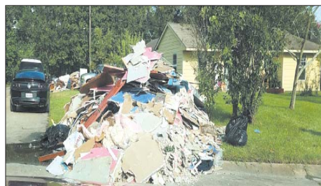
Flooded homes throughout East Harris county meant ripping out walls and floors, as seen at this house on Serpentine Street in Jacinto City near Hunting Bayou.
