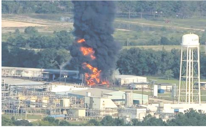
The Arkema chemical plant in Crosby had multiple fires and explosions, due to flooding and power failure of refrigerated chemicals.
