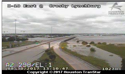
The I-10 bridge over the San Jacinto River was closed for most of the week due to high water and possible damage to the bridge.
