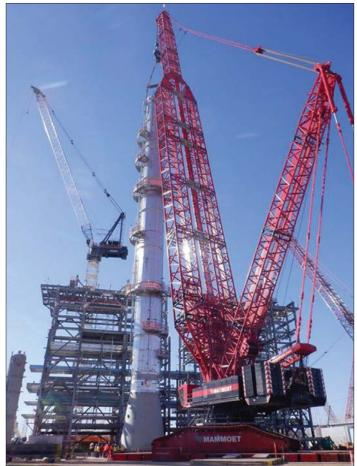
Large red cranes loom over LyondellBasell's Channelview site as installation of the company's propylene oxide, tertiary butyl alcohol plant's largest pieces of equipment, such as this 25-story-tall, 601-ton distillation tower are being installed. Once in operation, the PO/TBA plant will be the largest of its kind in the world.
