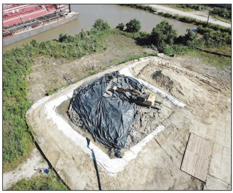
Excavation is taking place under a tarp or membrane, to contain the toxic material from being airborn.
