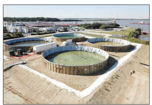
Four large open-air tanks are part of the destering process when water is encountered during the excavation work.
