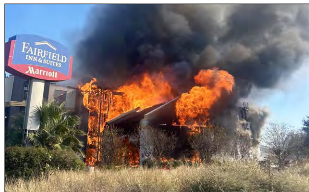
Four fire departments responded to the Fairfield Inn & Suites Hotel fire on the corner of Sheldon Road and I-10 on Thursday last week. Despite earlier attempts, the fire rekindled again on Friday and the building completely collapsed.
