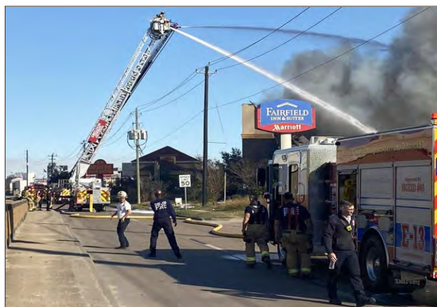
Four fire departments responded to the Fairfield Inn & Suites Hotel fire on the corner of Sheldon Road and I-10 on Thursday last week. Despite earlier attempts, the fire rekindled again on Friday and the building completely collapsed.
