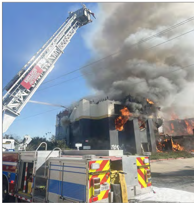
Four fire departments responded to the Fairfield Inn & Suites Hotel fire on the corner of Sheldon Road and I-10 on Thursday last week. Despite earlier attempts, the fire rekindled again on Friday and the building completely collapsed.
