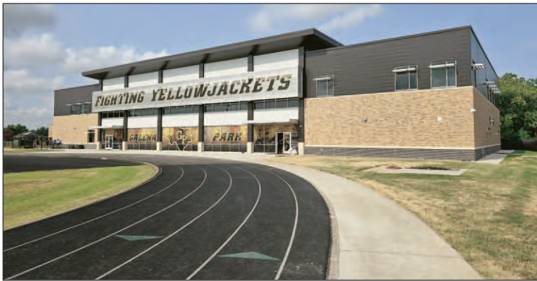
The new two-story field house at Galena Park High School is a state-of-the-art facility housing the Yellow Jackets football program. With an ever-growing program of 230 students this year, it couldn't have come at a better time.
